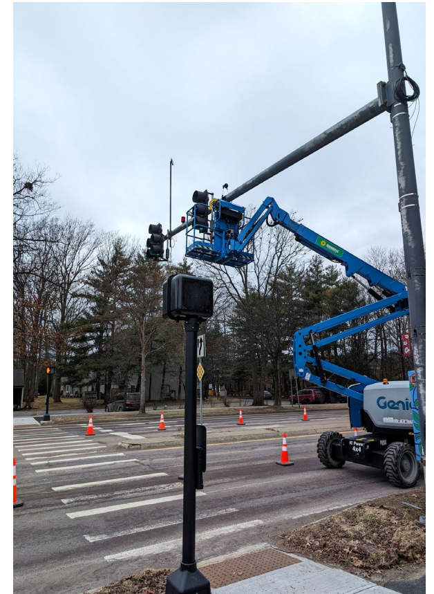
New Traffic Signal Installation on Dorset Street
